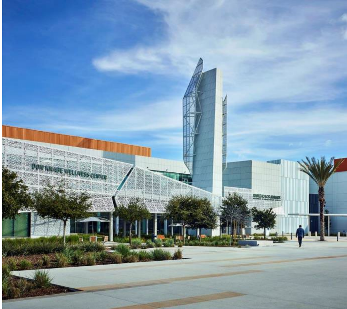
Project: Rancho Los Amigos National Rehabilitation Center; SmithGroup
